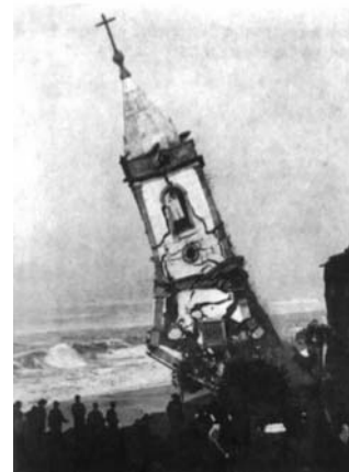
Figure 5. Holy Mary of Help Chapel destruction.
