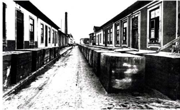
Figure 12. Concrete blocks construction.
