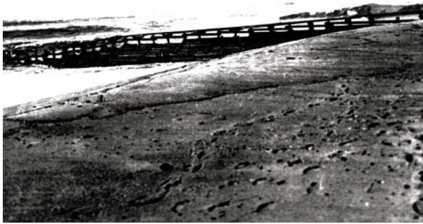
Figure 8. Experimental wood groyne.
