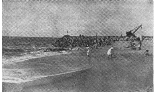
Figure 9. Groyne construction.
