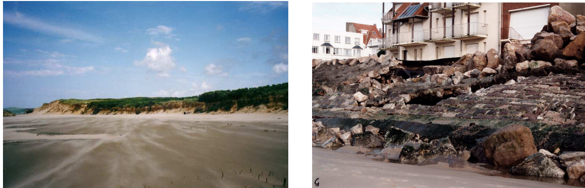
Figure 3. Some effects of the erosion in Wissant Bay: coastal dune retreat west of Wissant (photo M-H. Ruz) and Embankment collapse in Wissant in 2000 (photo P. Overlau)
