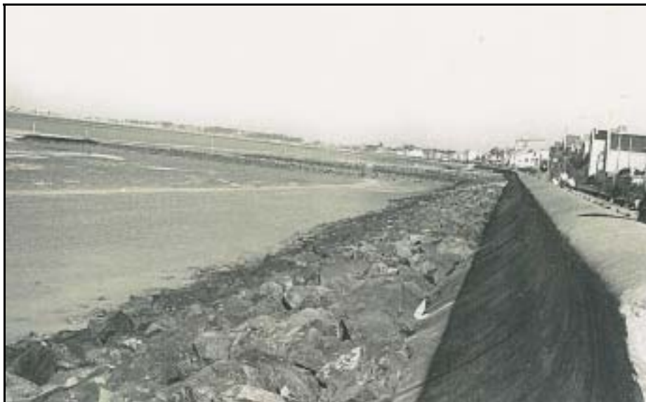
Fig.5: The beach prior to the beach-nourishment (1988). The foreshore is narrow, the groins and the rocks on the foot of the seawall are not efficient measures against erosion.
