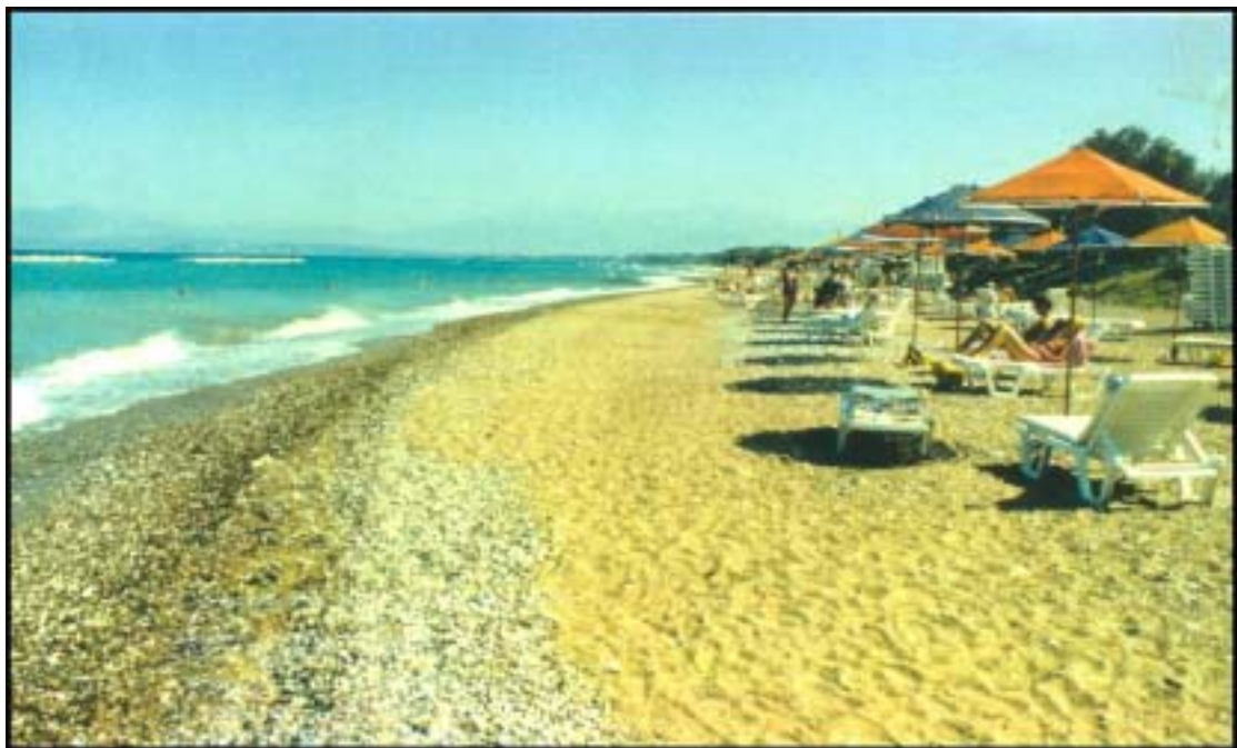
Fig. 9: East view of the beach after the construction of the breakwaters.
