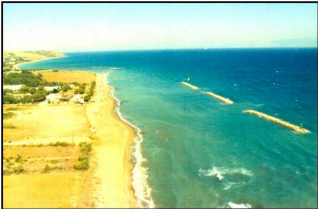
Fig. 7: View of the beach after the construction of the breakwaters.
