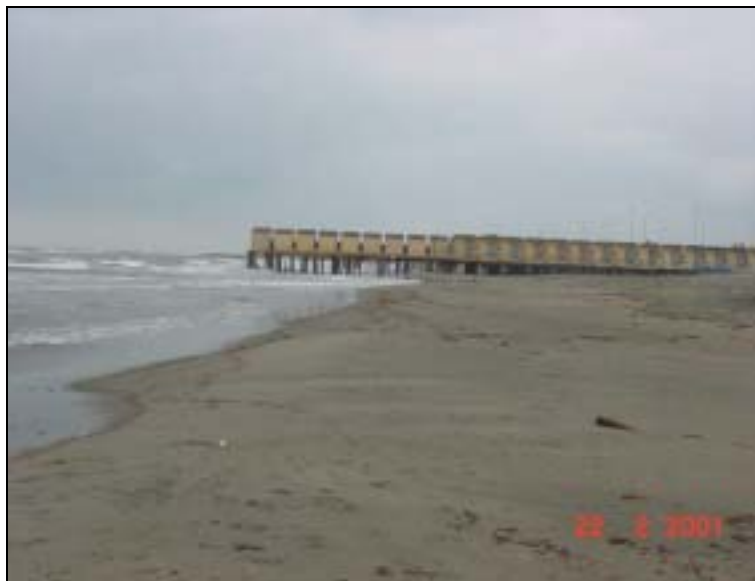
Fig. 9b: Section 3 (North) - Situation on 22 February 2001 (10 days after BMS installation).
