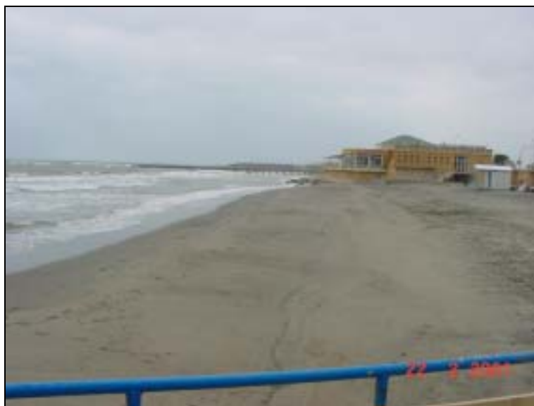
Fig. 8b: Section 2 (North) - Situation on 22 february 2001 (10 days after BMS installation).
