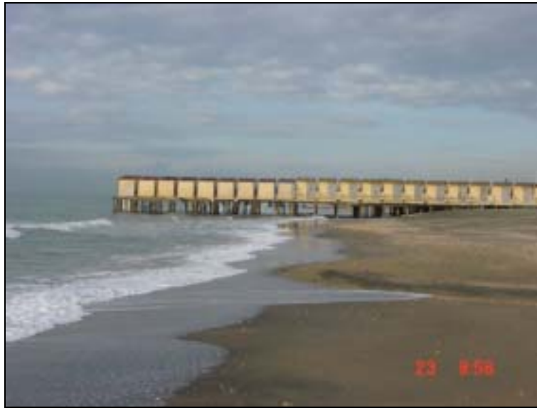
Fig. 9a: Section 3 (North) - Situation on 23 October 2000 (without BMS system).
