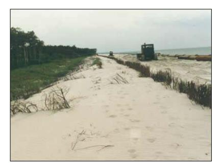
Fig. 28: Works over the renourishmened dune, pipeline is visible, Kuznica region, 1994 (photo by K.Furmanczyk).
