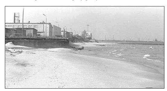
> Hard seawalls; constructing with concrete, using, when the erosion hazard is strong and the building are in direct danger (Fig. 26).
