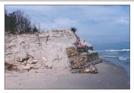
*Fig. 23: Seawall made with gabions lying over geotextil, Jurata, 1995 (photo by K.Furmanczyk)*
