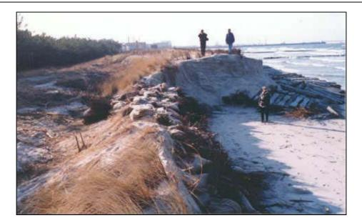
*Fig. 21: "Link-side effect", strong erosion behind the seawall in Wladyslawowo; combined seawall is visible as well as sacks filled with sand used for emergency coast protection during the storm, 1995 (photo by K.Furmanczyk).*
