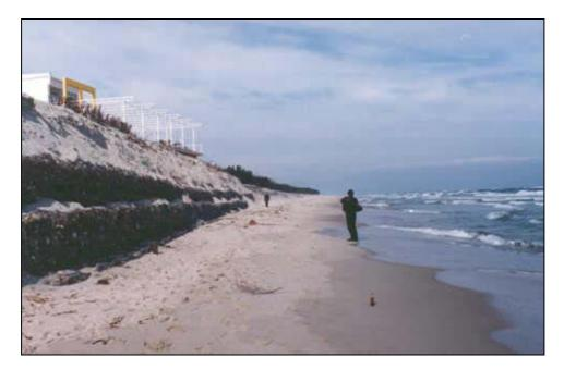
Fig. 22: Eroded dune, opened and visible gabion seawall, Jurata, 1995 (photo by K.Furmanczyk).
