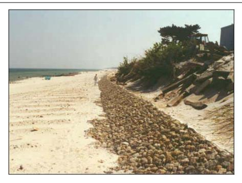
*Fig. 25: Gabions lying over the stony basis, seawall constructed in front of partly destroyed concrete's sleepers seawall, Kuznica, 1996 (photo by. K.Furmanczyk).*
