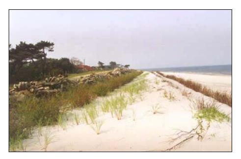
Fig. 18: Concrete's sleepers seawall, Kuznica region, 1992 (photo by K.Furmanczyk).
