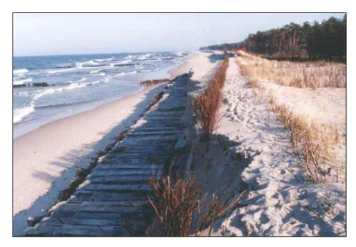
*Fig. 20: Structure of combined seawall visible after strong erosion of the protected dune, Wladyslawowo Harbour, 1995 (photo by K.Furmanczyk).*
