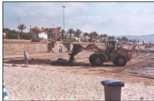
Fig. 12: Sand replenishment works (n°6)
