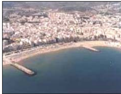
Fig. 8: Detached breakwaters (n°2)
