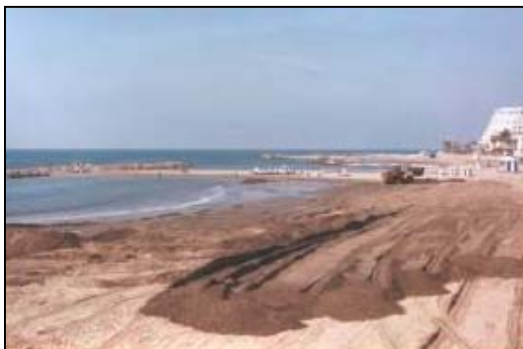
Fig. 11: Sand replenishment (n°6)
